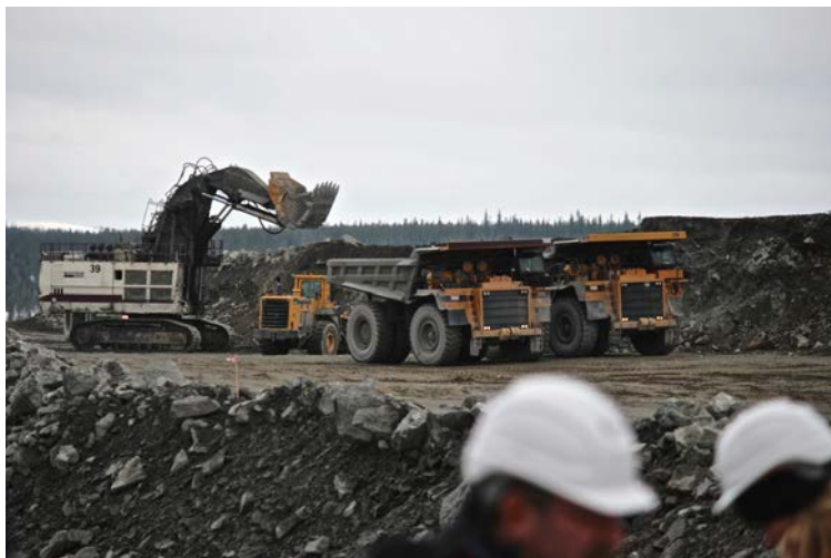
Haul trucks line up to take rock material from an excavator at Kovdorskiy.
