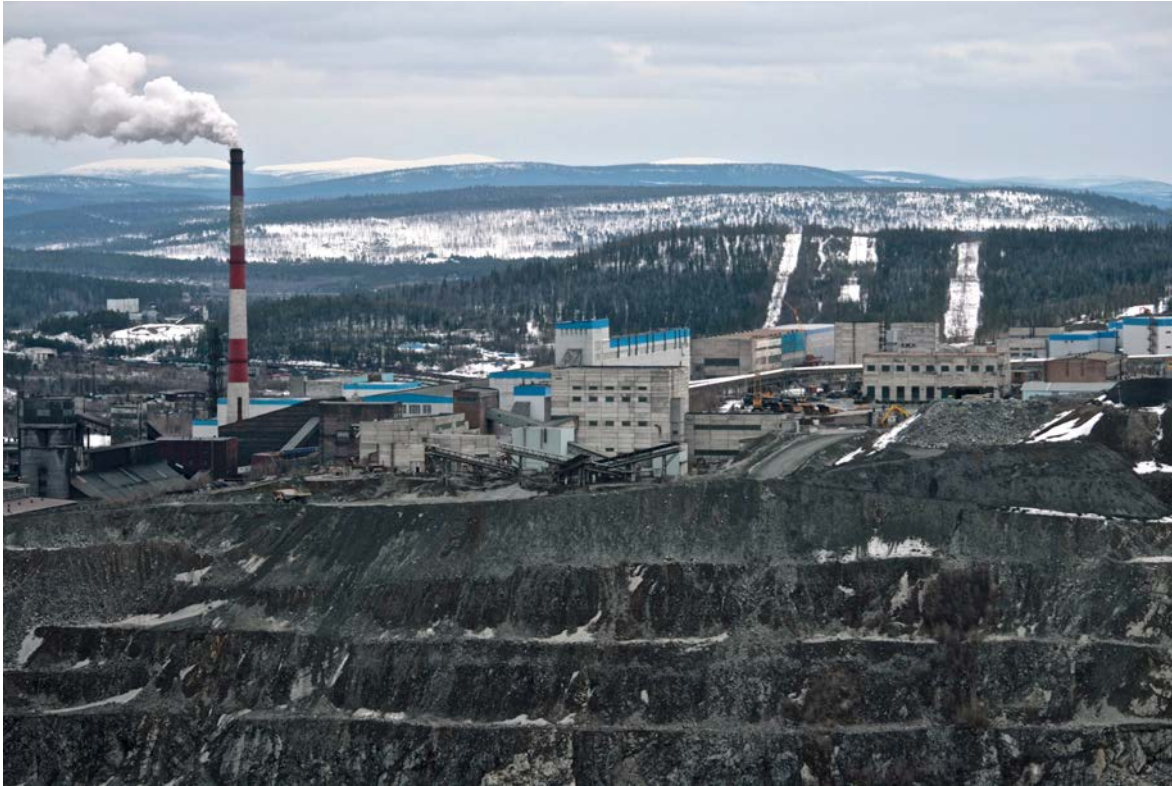
Processing facilities at EuroChem's Kovdorskiy phosphate and iron ore mine – the second largest apatite concentrate producer in Russia.
