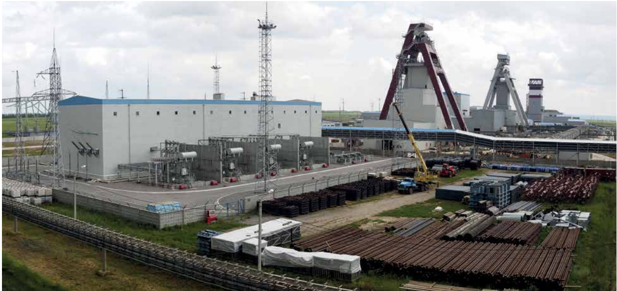
VolgaKaliy potash project - electrical substation and three shafts
